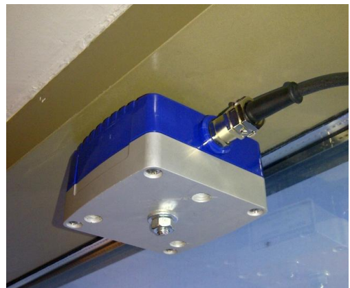
Geophone Mounted to the Ceiling
